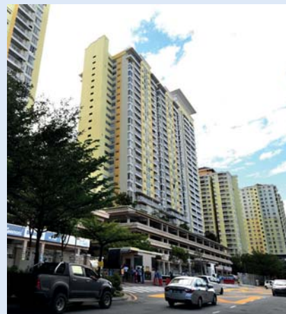
PV13 is one of the many landmark high-rises by Platinum Victory spread throughout Setapak
